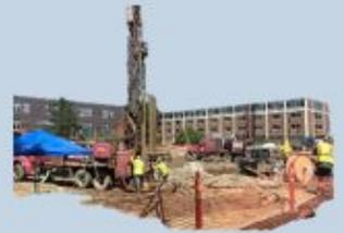
Two types of geothermal wells are installed on campus: horizontal wells are drilled under Bell Field, while vertical wells are drilled under the Bald Spot and the Mini-Bald-Spot. These wells will help with heating and cooling at Carleton.
