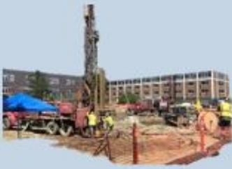
Two types of geothermal wells are installed on campus: horizontal wells are drilled under Bell Field, while vertical wells are drilled under the Bald Spot and the Mini-Bald-Spot. These wells will help with heating and cooling at Carleton.
